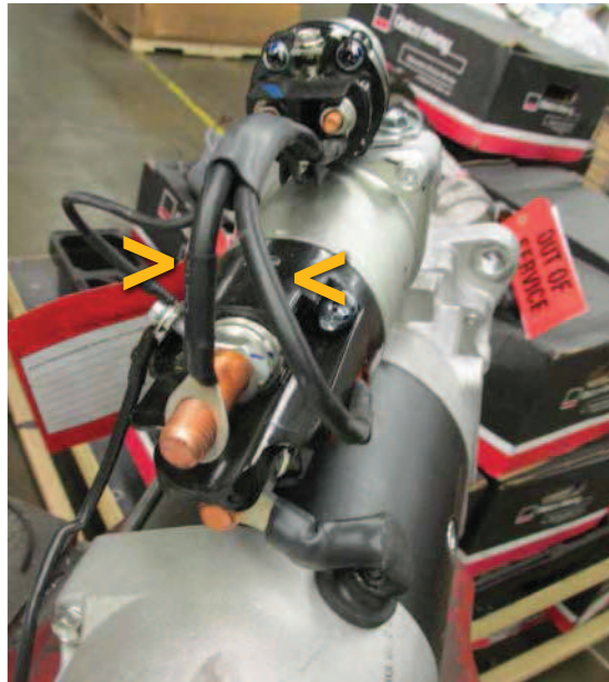
Sometimes these two wires will show heat damage "Puckering"
